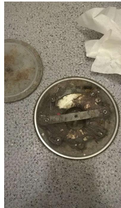
Fig 2: Shower drain with cover removed
